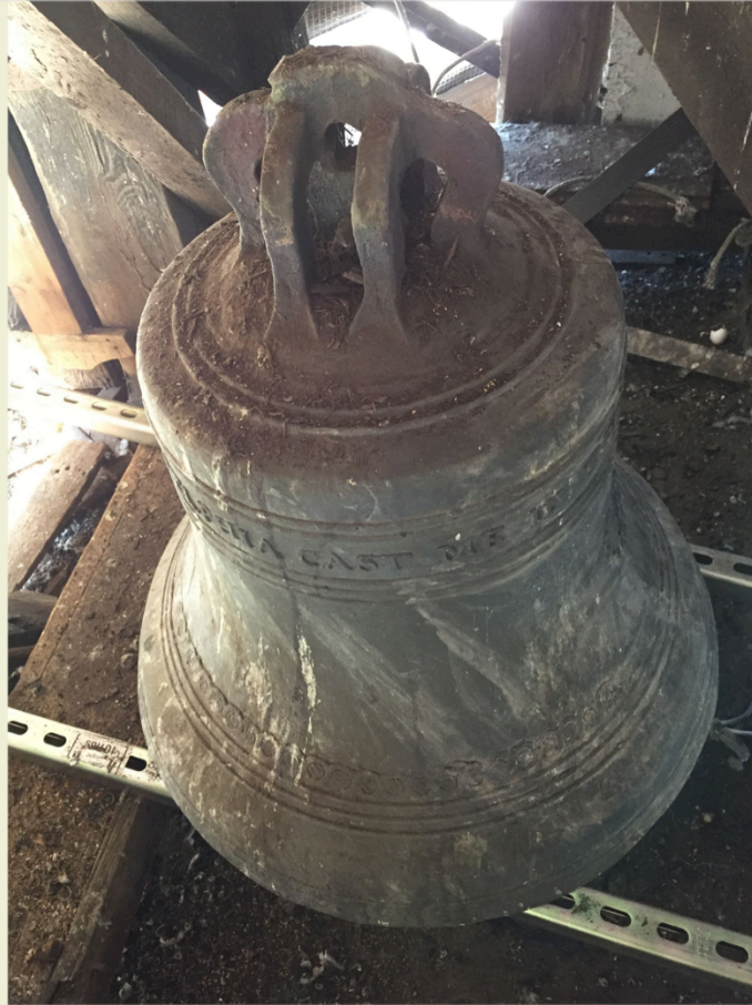
BELL PARTS FROM TOP TO BOTTOM: ARGENT, CANONS, CROWN, SHOULDER, INSCRIPTION BAND & INSCRIPTION, WAIST, MOULDING WIRES (TOP & BOTTOM) SOUNDBOW, LIP
